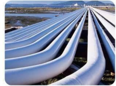
CROSS COUNTRY PIPELINE
